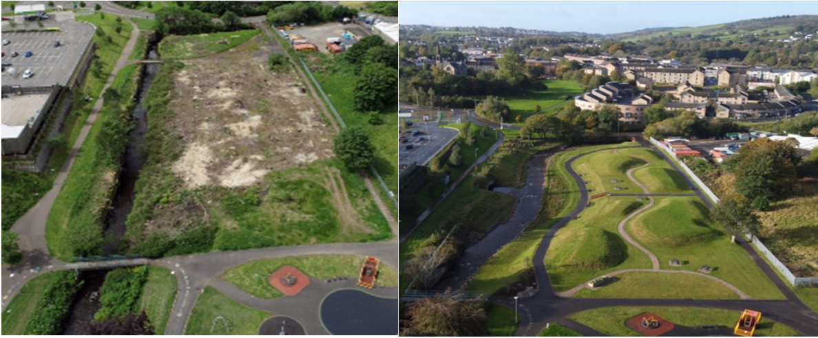
Figure 8: Lavern Water Restoration - Before and after restoration works (AmcoGriffen, 2024)
